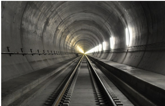
Feste Fahrbahn Gotthard Basistunnel (Faido-Bodio West).
